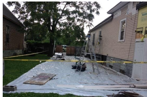
Lead-safe renovation prep with caution tape and plastic sheeting.
