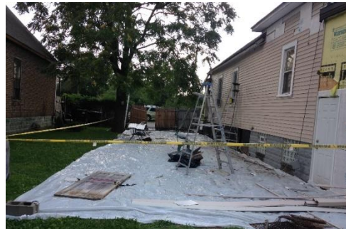
Lead abatement prep with caution tape and plastic sheeting.
