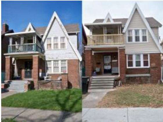
Before and after photos of a lead abatement project in Detroit.
