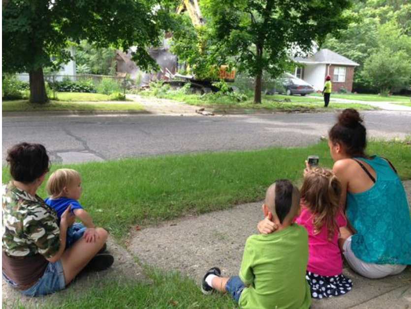
Dolphin Street residents, from left, Katie Pravic with her son, Corey Keegan, 2, seated on her lap; Dezmond Belanger, 5; Nevaeh Belanger, 4; and the Belangers' sister, Shawna Hansen-Ross, watch a city-contracted crew demolish a house across the street from their neighboring homes. Pravic and Hansen-Ross said they received no notification of the impending demolition, or information on keeping the children indoors and safe from lead dust pollution (Photo: Keith Matheny/Detroit Free Press)
